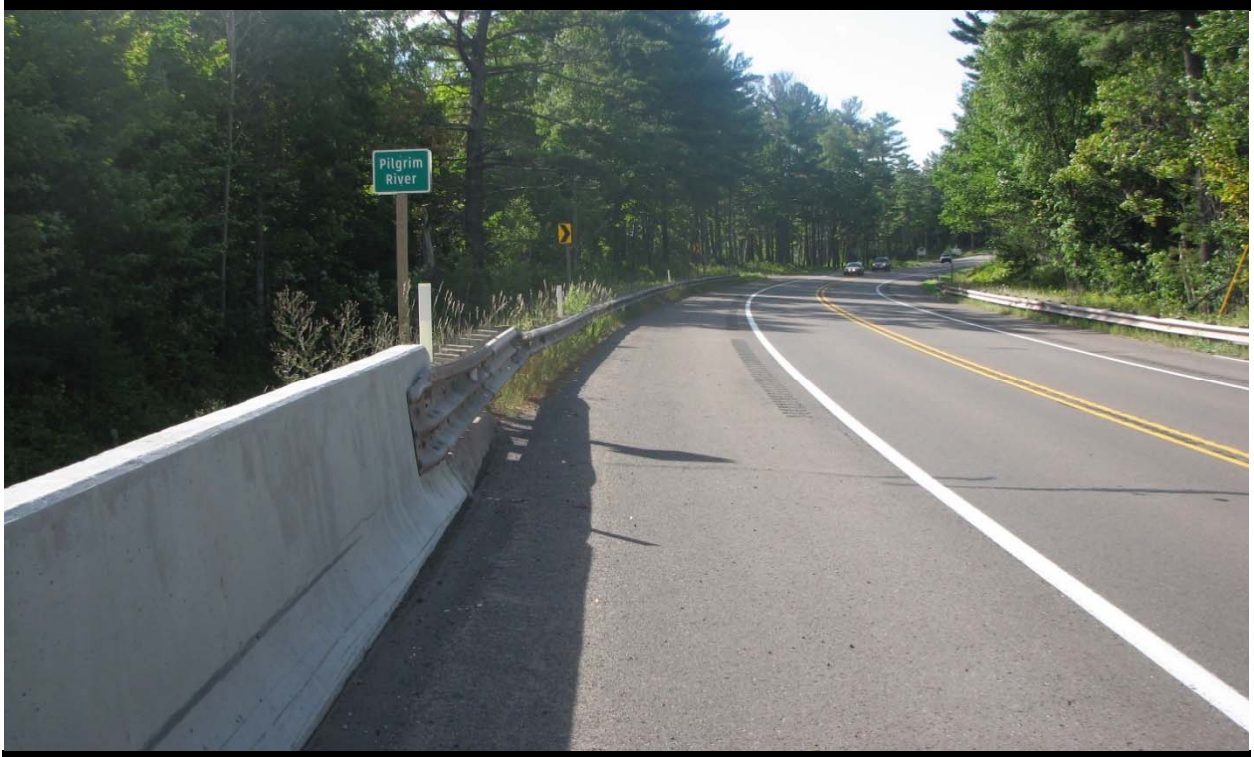
Figure 4 The condition of the roadway and embankment can help identify distress within a culvert below. Characteristics to inspect include the pavement, guardrail, shoulders, slope stability, and embankment erosion.
