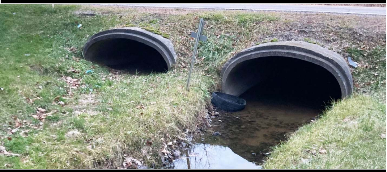
Figure 8 Concrete barrels should be checked for cracking, spalling, deterioration, joints, alignment, and infiltration and exfiltration (photo: Kent County Road Commission)
