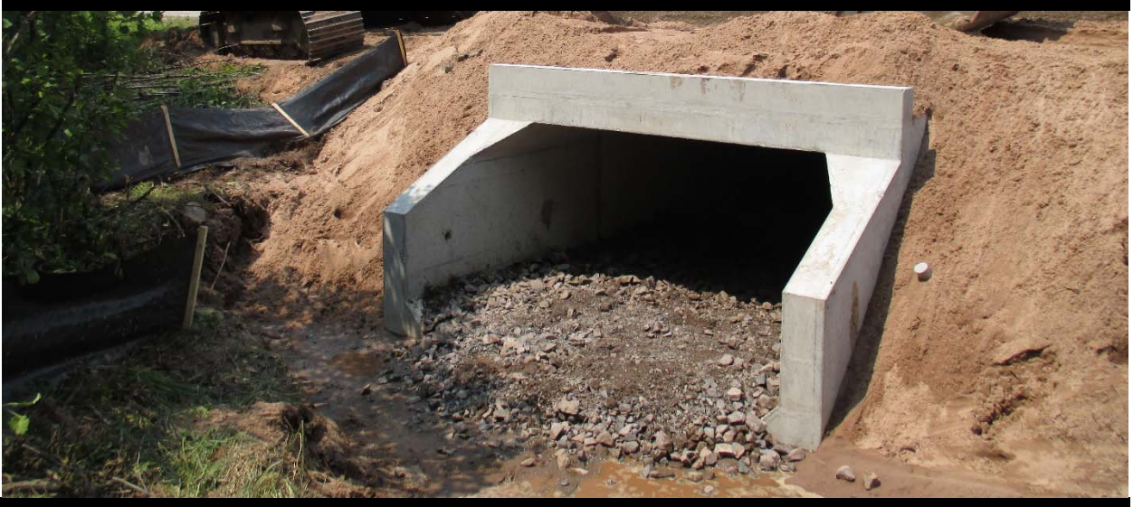
Figure 6 End treatments are designed to protect the culvert barrel and surrounding area from erosion and seepage. Concrete end treatments are checked for cracking and surface damage. Metal treatments are inspected for deformation and corrosion. Additionally, end treatments should be evaluated for scour and stability and for settlement and rotation.
