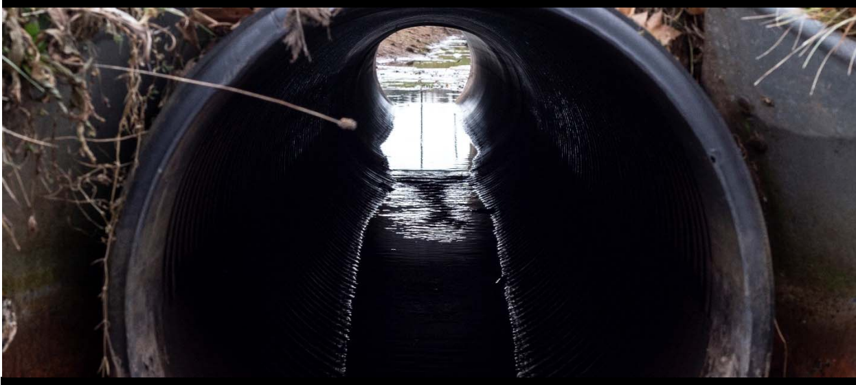
Figure 7 Plastic barrels need to be checked for changes to their cross-sectional shape, surface damage, local buckling, joints, alignment, and infiltration and exfiltration.
