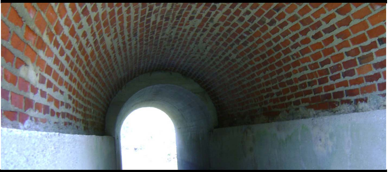
Figure 10 Masonry barrels are checked for movement of masonry units, mortar, and efflorescence (photo: St. Clair County Road Commission)
