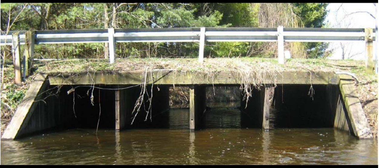
Figure 11 Timber barrels should be checked for connections and missing members, decay, checks and shakes, structural cracks, delamination, abrasion and impact, and distortion (photo: Fleis & Vandenbrink Engineering)
