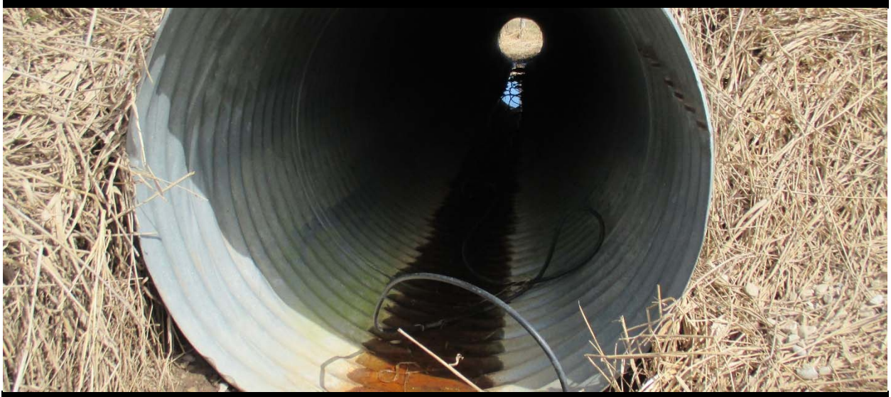
Figure 9 Corrugated metal barrels are checked for surface damage, corrosion, abrasion, shape, joints and seams, alignment, and infiltration and exfiltration
