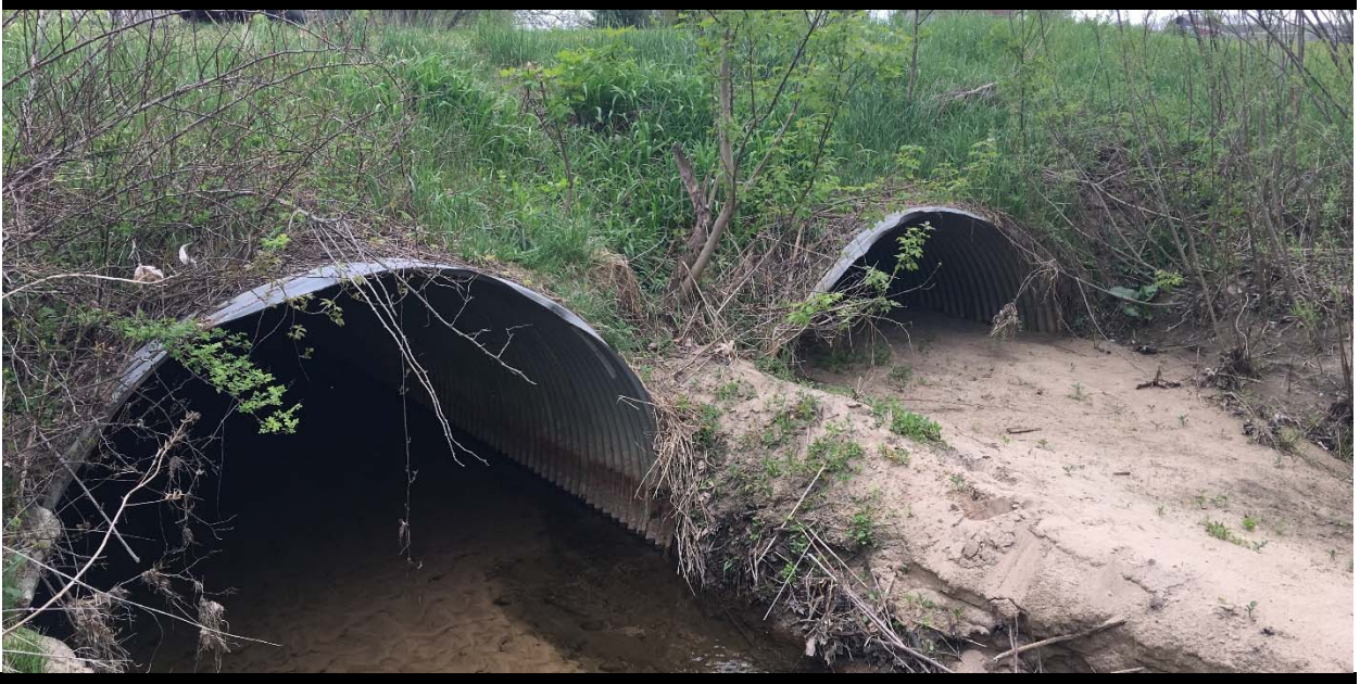
Figure 5 Culvert placement can cause damage to the area around the culvert due to scour or ineffectiveness due to blockage. The characteristics to inspect include channel alignment, bank erosion & scour, existing scour protection, and blockage.
