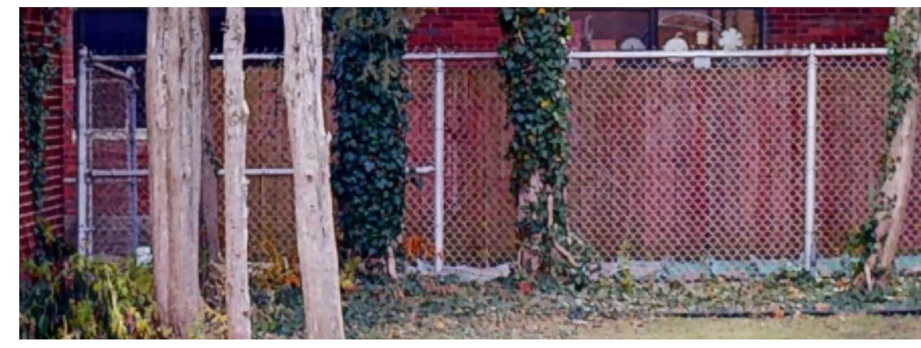
EXISTING 6 FT HIGH CHAIN LINK PERIMETER FENCE
